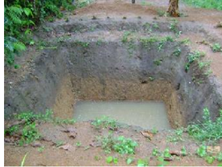
WCP when constructed
